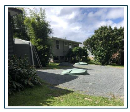
Photograph 8 – Looking south at the existing OSMS on No. 9. The absorption trench for the southern tank runs parallel to slope from the tank past the tree and shed (background). The absorption trench for the northern house runs from the tank under the gravel and lawn in the foreground.
